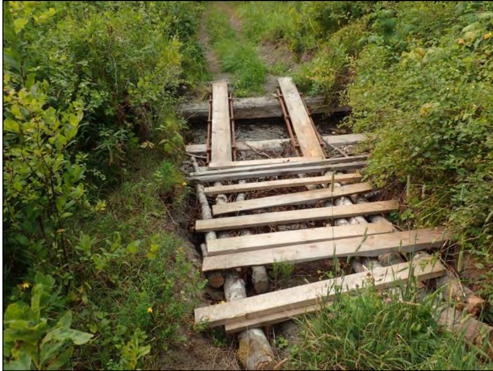
Plate 5.1-4. Temporary bridge used by ATVs along the old rail trail between Hills and Summit Lake. Bridge crossings will need to be improved following appropriate authorizations.
