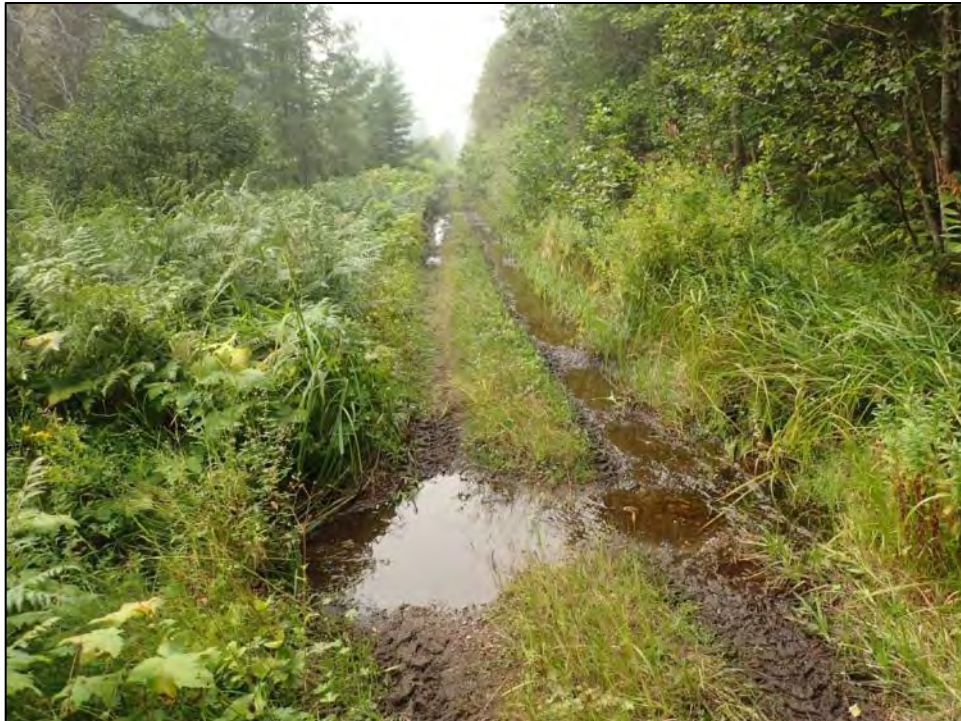
Plate 5.1-3. Section of the old rail trail between Hills and Summit Lake where water is currently pooling and drainage improvements are needed.
