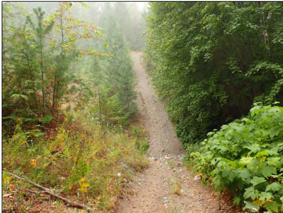
Plate 5.1-1. Steep section of rail trail near the gravel pit which a geotechnical review recommended is re-aligned and culverted.
